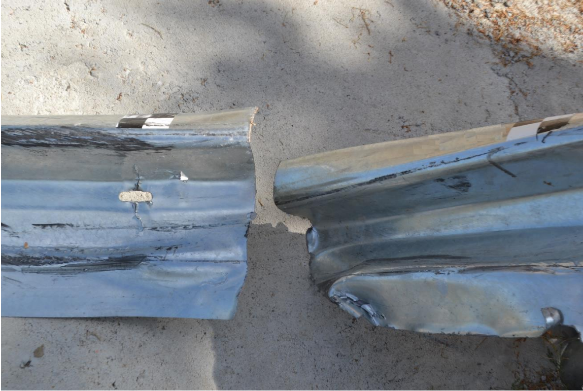
Figure 87. Rail Rupture from 2270P Impact
